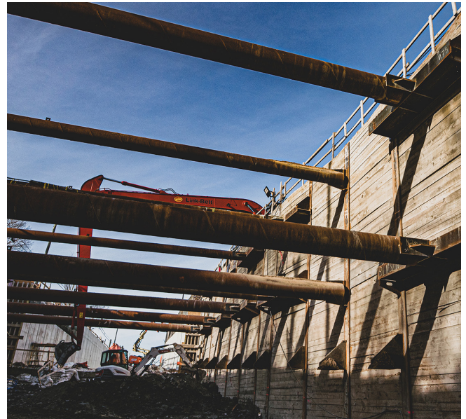
Photo: Humber College portal excavation.
