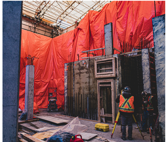
Photo: Survey work in the Finch Station main entrance box.
