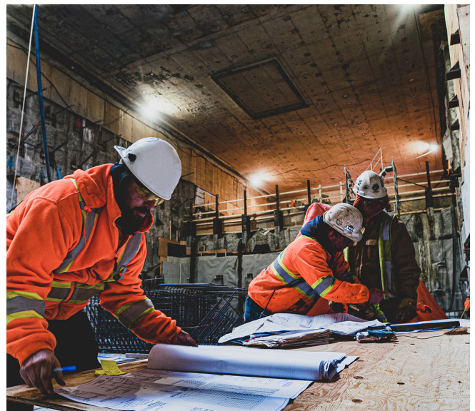
Photo: Finch West station crews review drawings in the main station box.
