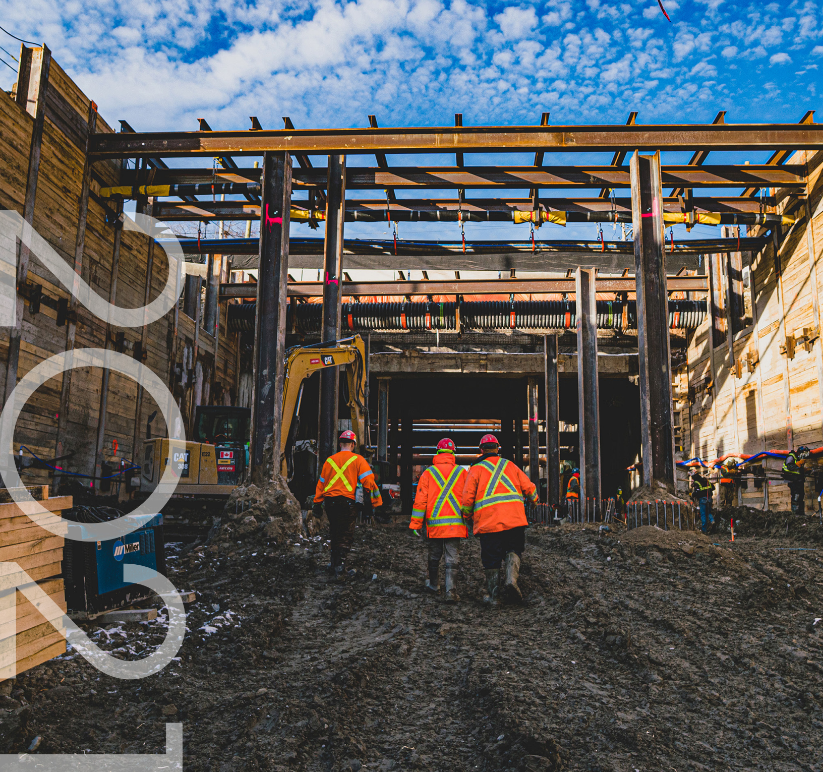
Photo: Humber College Station, view north under Humber College Boulevard.
