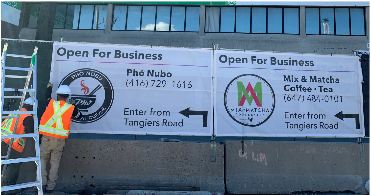
Photo: Good Group (a non-for profit agency providing employment opportunities to local trades) team members, hang signage banners to help local business during construction of the Finch West Light Rail Transit project at the corner of Finch Avenue West and Keele Street.
