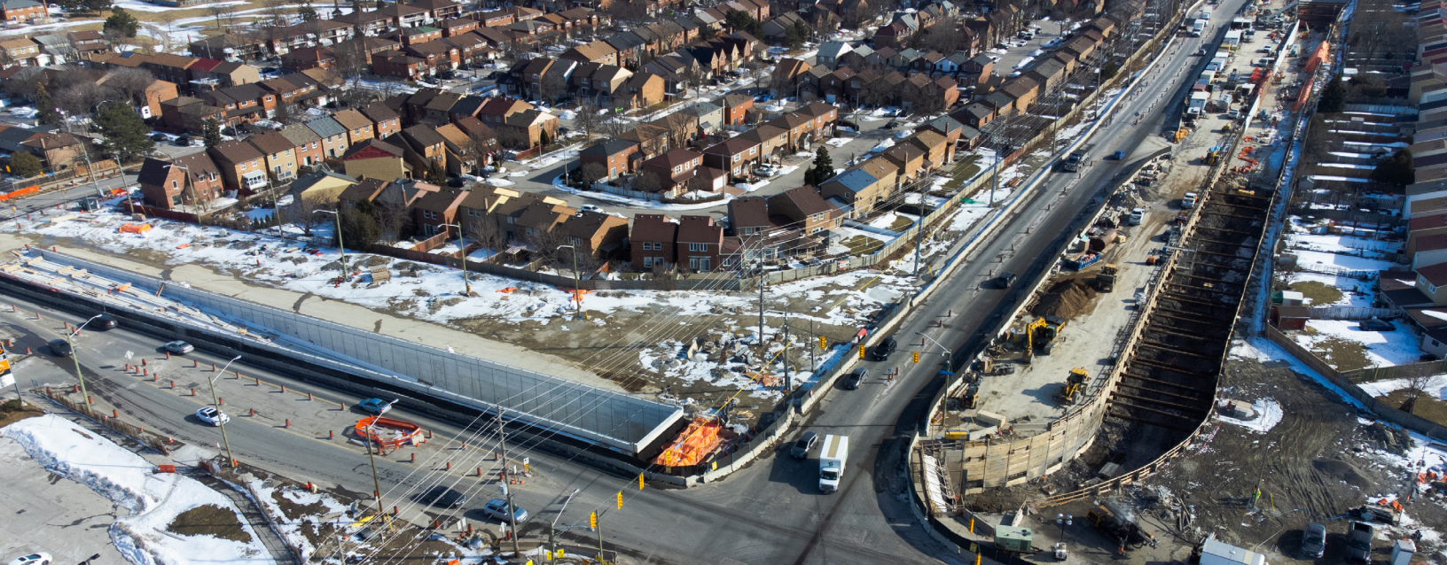
Photo: Humber College entrance portal running under the intersection of Highway 27 and Finch Avenue West.
